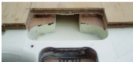
For the very first pass we used a 3/8" router bit and cut only to a one-third depth
