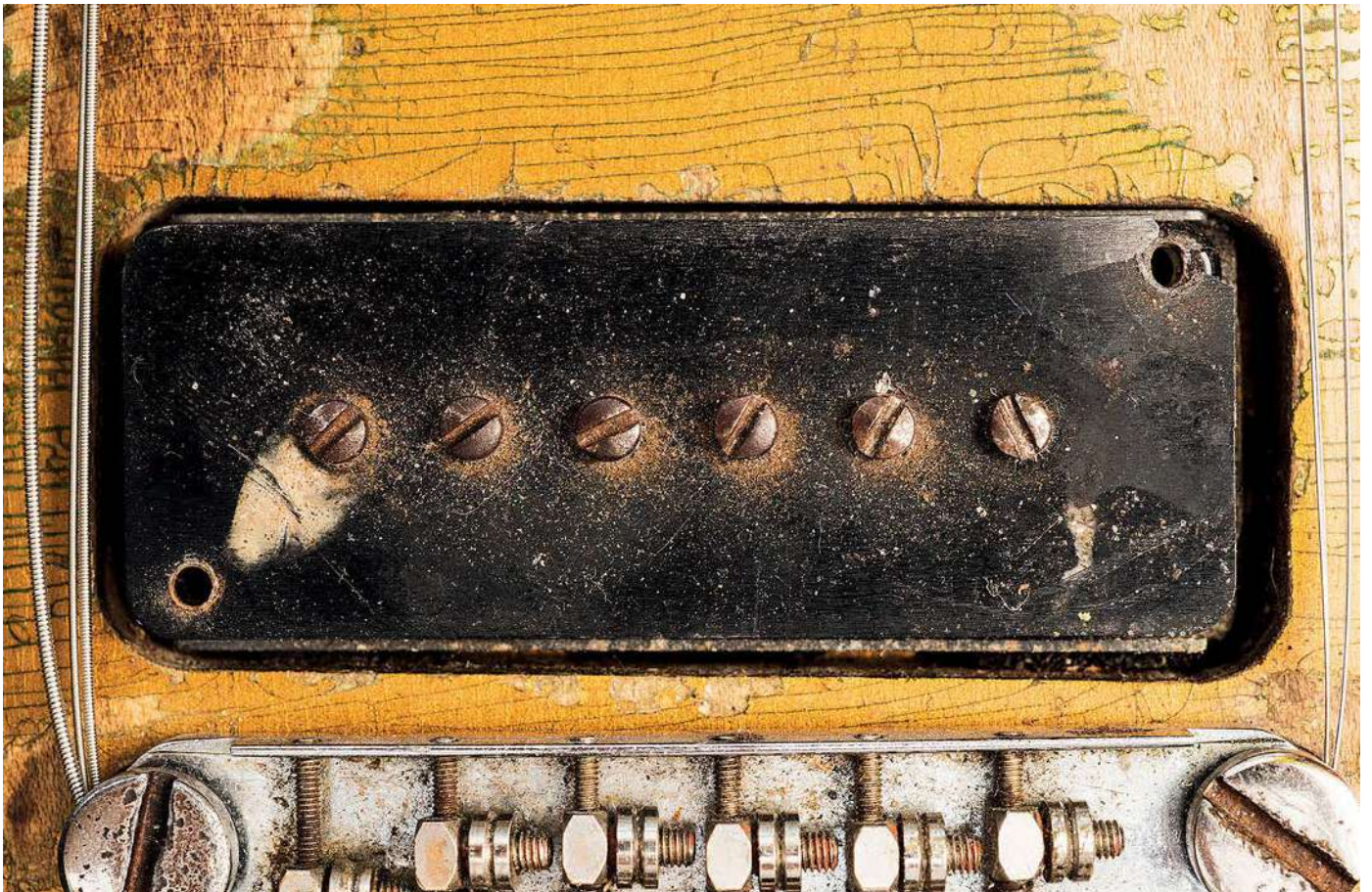
BELOW The diagonal screw holes on the bridge pickup show how Gibson was still working out the best way to do things at this early stage
